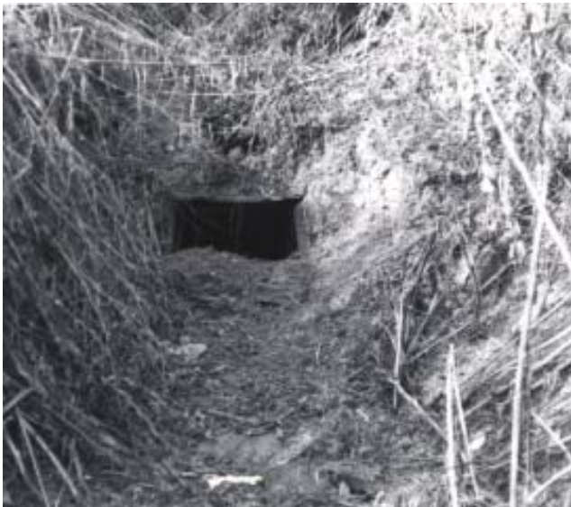
The Boardinghouse Tunnel in the Adams Canyon area of Santa Paula oil field, dug over 100 years ago, as photographed in February 1980. The tunnel is one of 26 Adams Canyon oil tunnels dug by Union Oil Company (or by companies that eventually merged to form a part of Union Oil).
