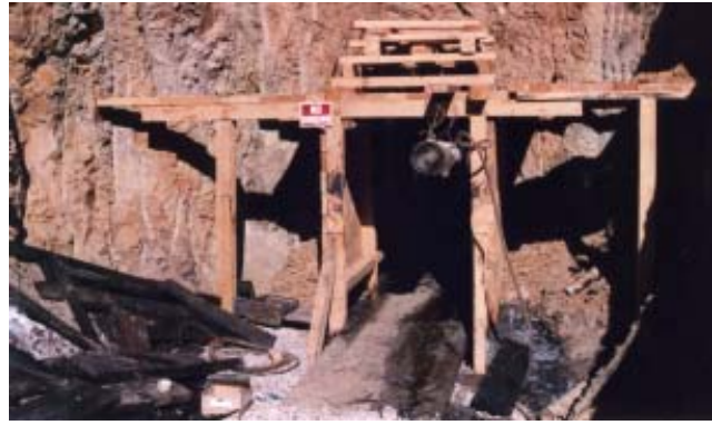
Mouth of the Boardinghouse tunnel as it was plugged and abandoned in 1997. The oil tunnels slanted slightly upward as deep as 400 feet into the sharply tilted strata of Sulphur Mountain, which rises abruptly north of the present City of Santa Paula. In the 1860s the tunnels produced more oil in California than any other production method. Photo by P. Kinnear.
