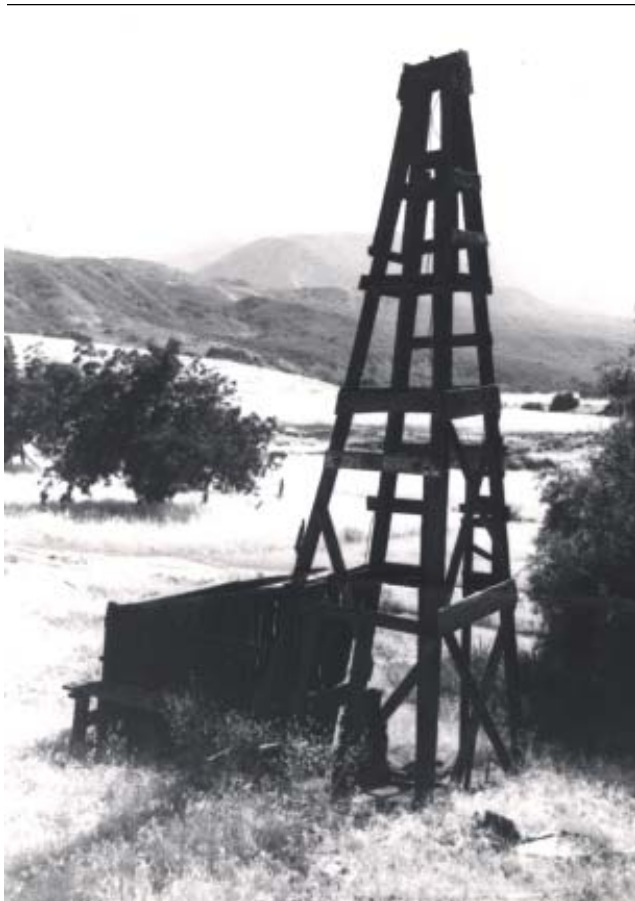
Remnants of the activity of California's early oil pioneers still dot the landscape. Natural oil seeps abound in this region of central Ventura County.
