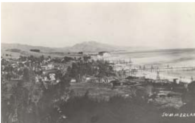
Summerland oil field, Santa Barbara County, around 1900. Onshore drilling started here in 1886. As field development continued, operators realized the oil sands extended under the ocean. To reach the offshore sands, piers were built over the water to support drilling and production machinery. The piers, though faint, are seen in this photo.
