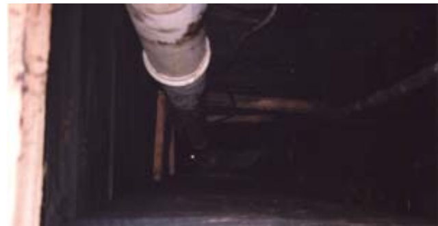
Inside the Boardinghouse tunnel during plugging and abandonment procedures in 1997. Completed tunnels generally were about five feet high and no more than four feet wide. Miners who made the tunnels chiseled out a gutter on the tunnel floor, lining it with redwood planks. Because of the steep grade, oil and water flowed easily down the gutters, out of the tunnels, and into the holding tanks. The airpipe was installed temporarily during abandonment operations. Photo by P. Kinnear.
