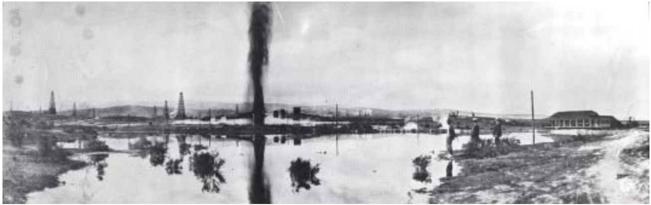
This was the greatest gusher of them all, the famed "Lakeview Gusher" near Maricopa, Kern County, in 1910. The well, "Lakeview" 1, spewed oil and sand for 18 months before it finally quit, producing over 8 million barrels of oil, an amount equaling about 10 days of California oil production in 2001.
